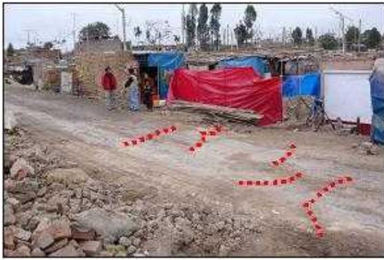
Figure 3. Ground tension cracks
