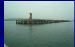
Breakwaters are constructed to maintain the calmness of the basin and ease of handling of cargo at quay walls. To perform these aims, breakwater should be designed to be safe against strong wave forces and to cut the transmission of wave forces.
