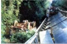
A bridge on the road from Siem Reap City to Banteay Srey temple was destroyed on April 10, 2004 following the passage of a convoy of heavy trucks carrying timber.
