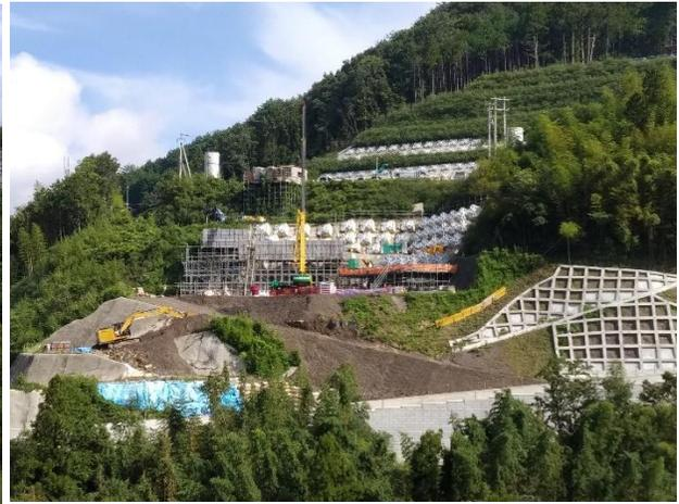
Figure 13 the slope protection on the abutment
