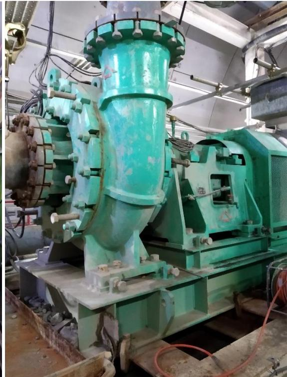
Figure 5 pump for drain slurry out
