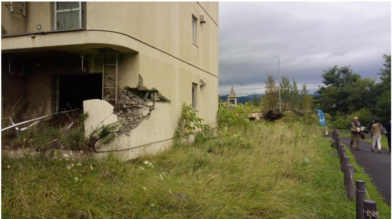
Fig.42. a damage caused to the building by the bridge due to volcanic mud / the bridge can be seen ahead
