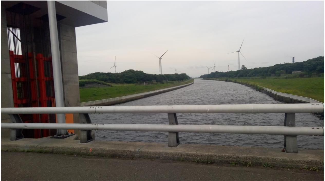
Fig.27. Ishikari River Gate and windmills supplying energy to facility
