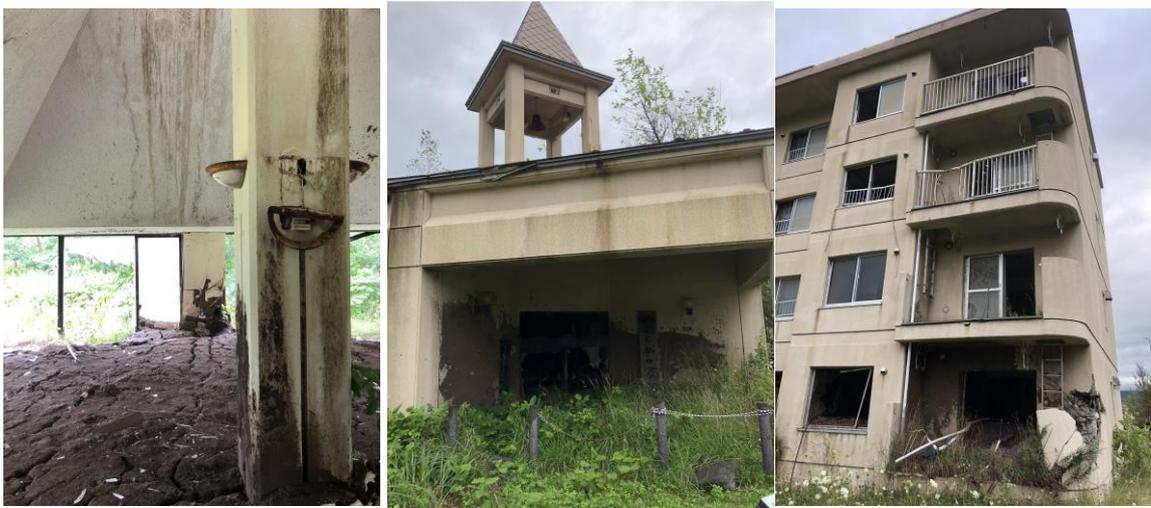
**Fig16.** Raw scars of damaged by the eruption
