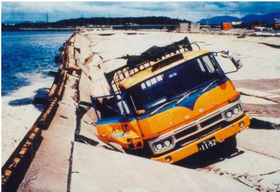
Fig.3 Damage to a sheet pile quay wall at Akita port during 1983 Nihonkai-Chubu earthquake (After Akita prefecture)
