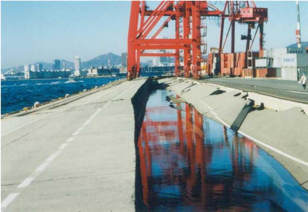
Fig. 5 Damage to a caisson quay wall at Kobe port during 1995 Hyogoken-Nambu earthquake
