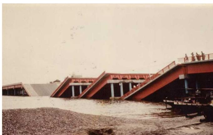
Fig. 2 Damage to Showa-Ohashi bridge due to liquefaction during 1964 Niigata earthquake
