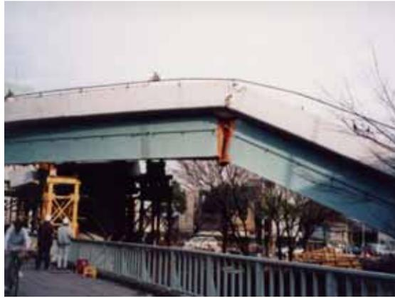
Photo 2. Collapsed bridge (1995 Hyogo-ken Nanbu Earthquake).
